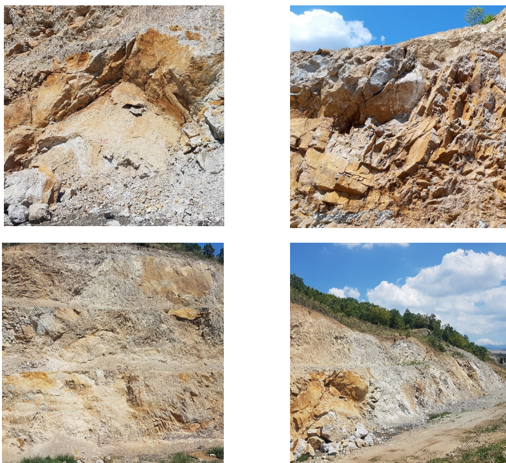
Figure 1. Appearance of a local rock fall (left up), typical picture of relatively fresh jointed andesite (left right), typical picture of altered andesite (down left) and a view on fault zones with higher level of alteration (down right).
