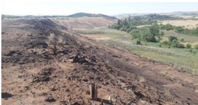
Figure 2. Downstream slope of the side tailings dam constructed of cycloned sand for TSF5, TSF6 and TSF7
