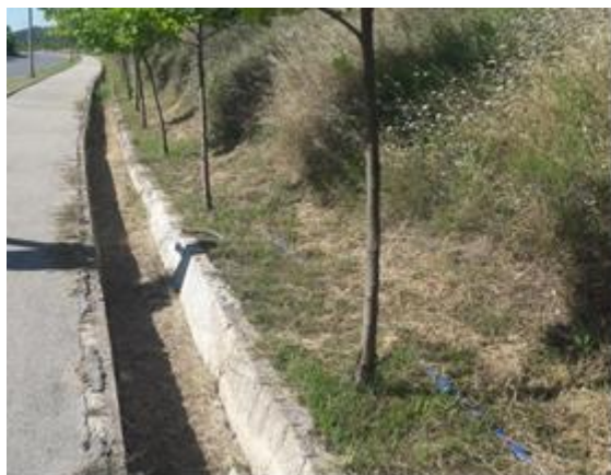
Figure 1. Concrete stormwater channel from Probištip, within the TSFs 5 area
