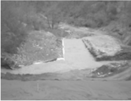
Picture 14. Drainage carpet in the final situation
