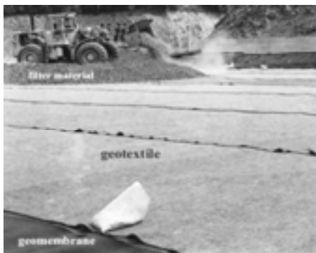
Picture 10. Lining of filter material
