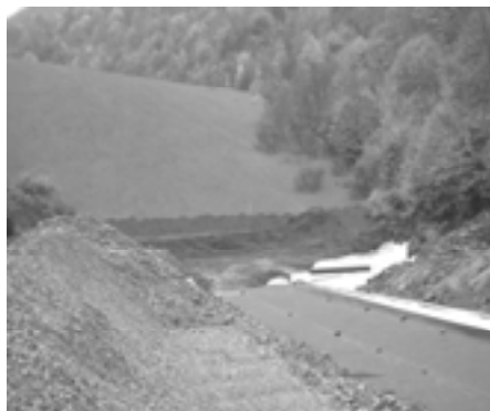
Picture 12. Construction of drainage carpet
