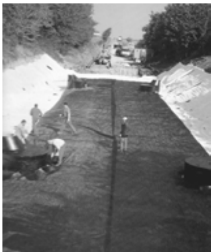
Picture 6. Lining of bottom drainage layers
