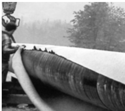
Picture 9. Lining of drainage pipes with geotextile
