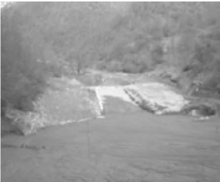
Picture 15. Drainage carpet in exploitation
