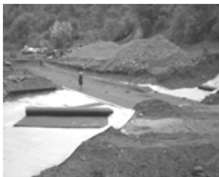
Picture 13. Construction of drainage carpet
