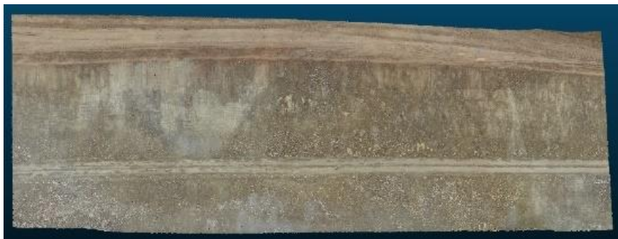
Fig. 10. First survey on 13.12.2022
