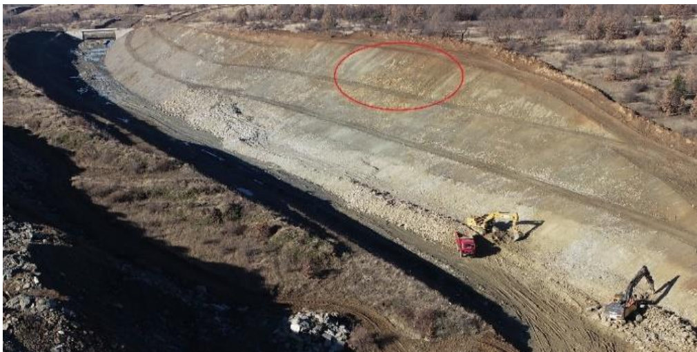
Fig. 3. Landslide condition on 27.09.2023
