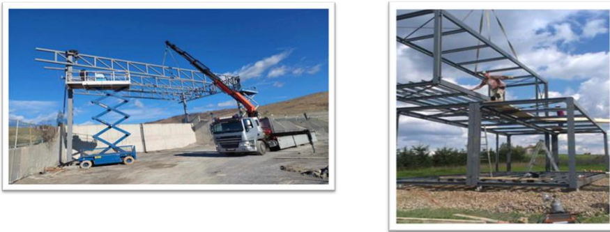
Fig.4 Assembling the steel components.
