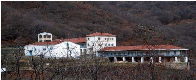
Figure 2 – Current state of the monastery
