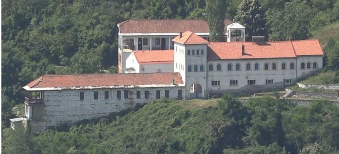
Figure 3 – Current state of the monastery
