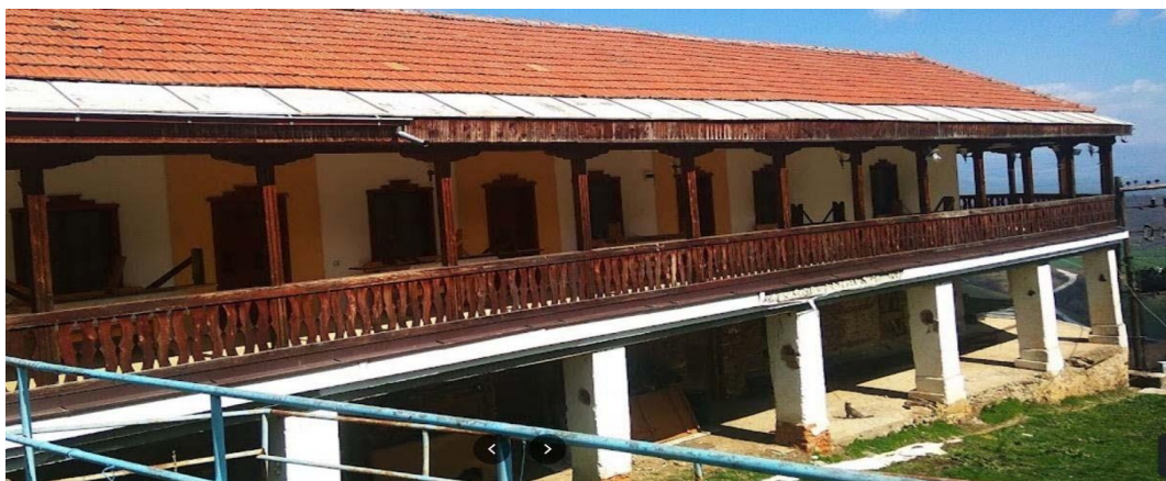
Figure 6 – Current state of the monastery
