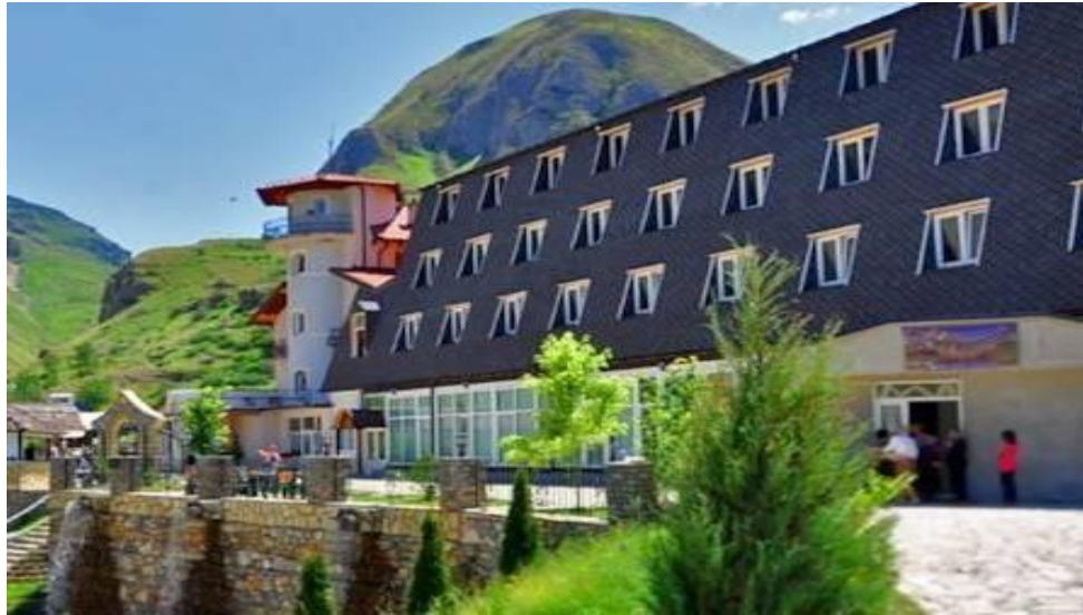
Figure 2. Argena Ski Center in summer
