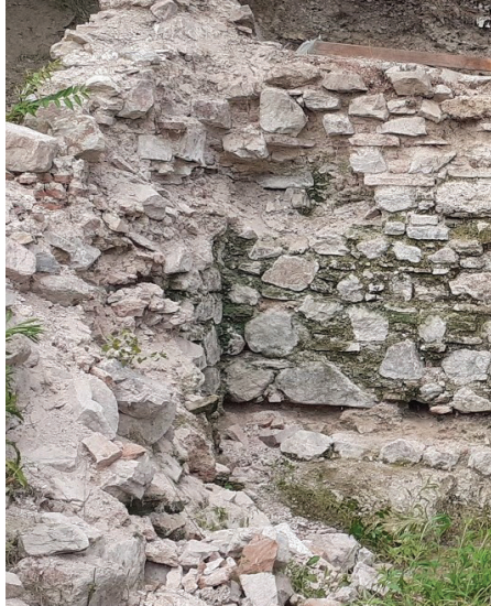
Fig. 6. Detail of construction technique opus incertum on the west wall.
