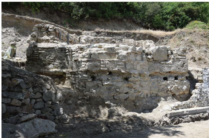
Fig. 2. Detail of the construction technique Semi opus cloisonné cum lignum on the east wall.
