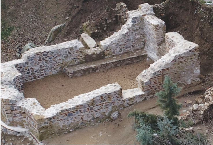
Fig. 11. North wall of the medieval church after conservation and restoration.
