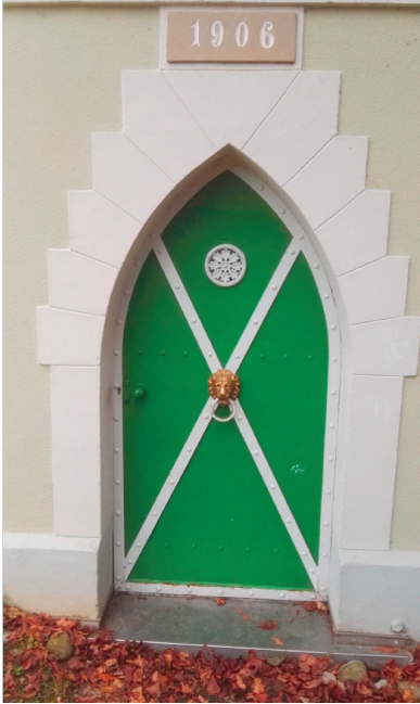
Fig. 6: Entrance door to water storage in Schlatt unter Krähen (photo by author)
