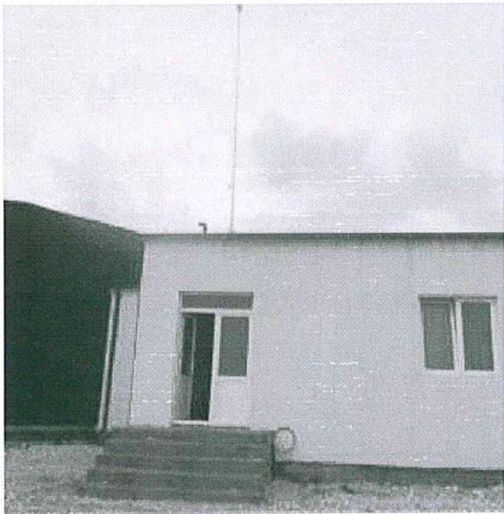
Figure 4. Provectron S6.60 on the roof of the machine room (Picture taken by author 1 )
