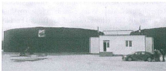
Figure 3. View of part of the biogas power plant in Porodin (digester and machine room) (Picture taken by author 1 )
