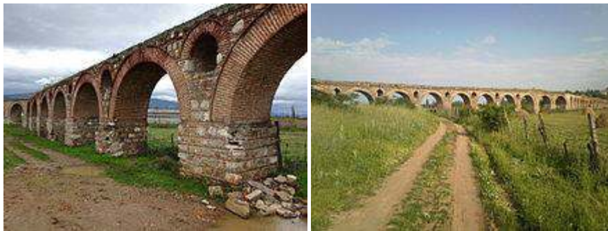
Figure 2. Skopje Aqueduct (Junist Aqueduct).
