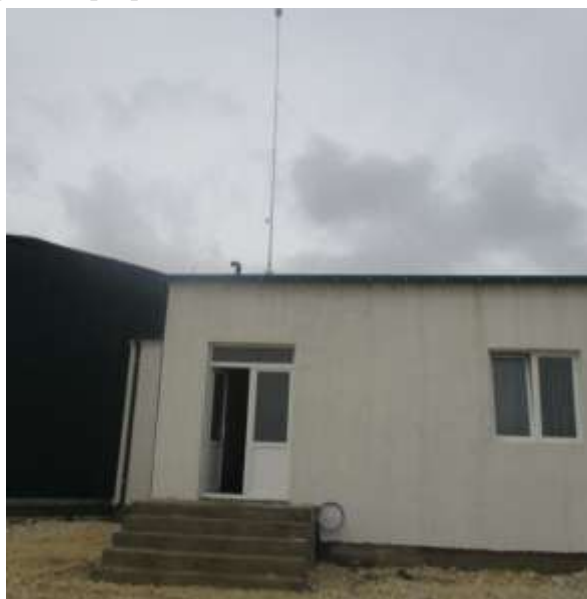
Figure 4. Provectron S6.60 on the roof of the machine room (Picture taken by author 1 )
