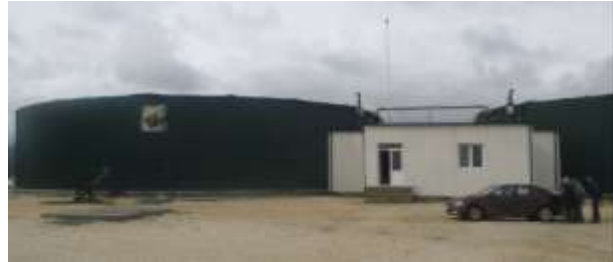
Figure 3. View of part of the biogas power plant in Porodin (digester and machine room) (Picture taken by author 1 )
