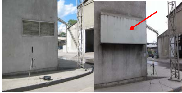
Figure 8. Cement mills` compressor station
