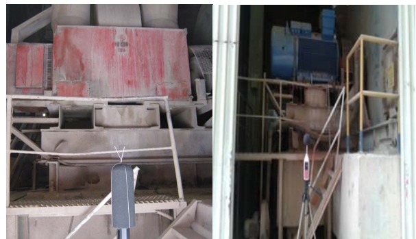
Figure 4. New Exhaust fan for rotary kiln 4
