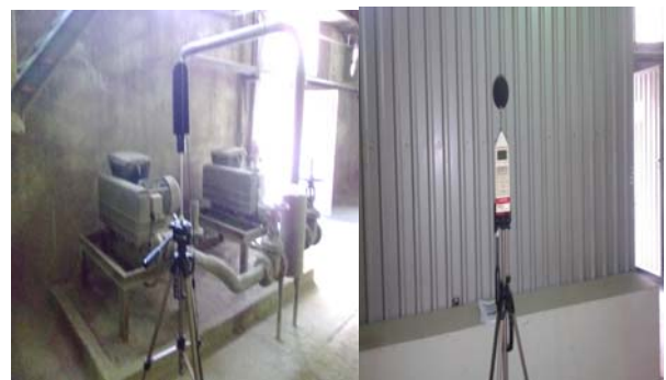
Figure 3. Closing blowers in an acoustic enclosure
