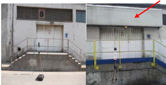
Figure 7. The compressor station in solid fuel preparation facility
