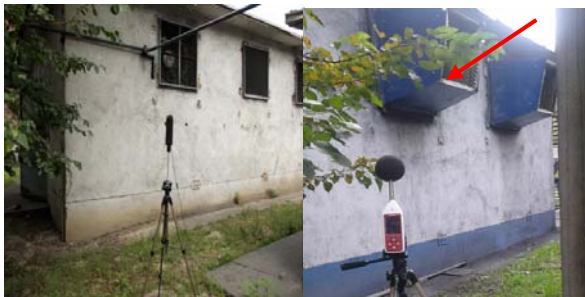
Figure 6. The compressor station in solid fuel preparation facility
