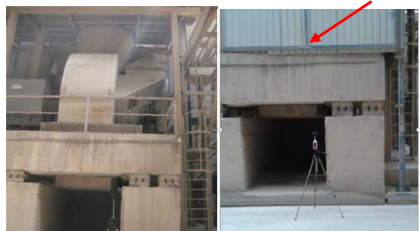
Figure 5. Fencing of exhaust fan for kiln 3
