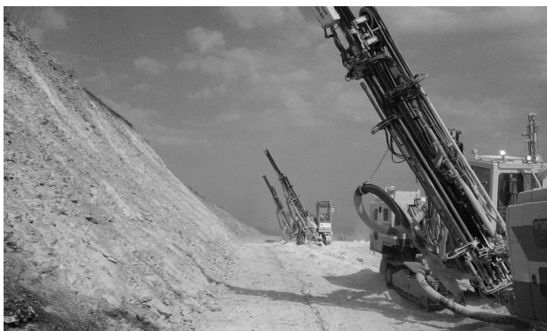
Photo 1: The drilling process of the contour drillings
