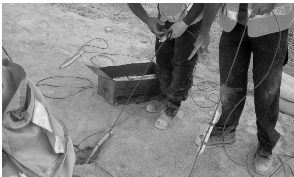
Photo 5. The procedure of filling the contour drilling
