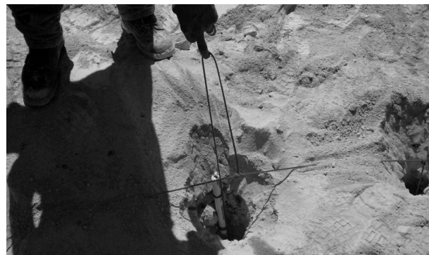
Photo 6. The length of the yarn pulled by holding the finger shows the distance of 0.6 [m] that remains without filling the top of the drilling
