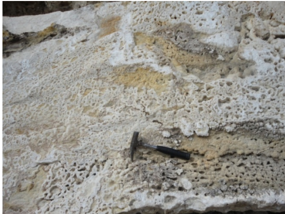
Figure 2. Stratified, porous and cracked light grey travertine
