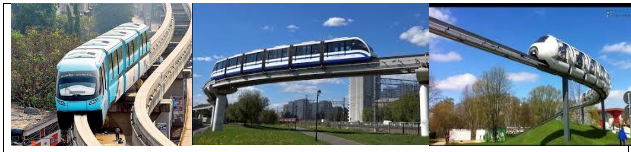
FIGURE 1. STRADDLE TYPE OF MR STRUCTURE
