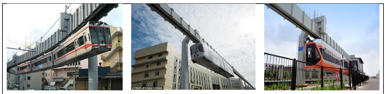
FIGURE 3. SUSPENDED TYPE OF MR STRUCTURE
