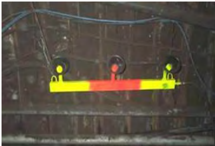
Figure 3: Example of installation of the triplets of respirators in the side of the roadway.
