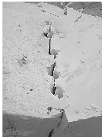
crack between new part of block
