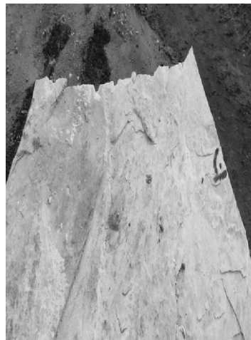
broken new part of block
