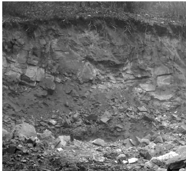
Picture 2. Cross-section of the incline of the terrain with structural deformities and existing cracks
