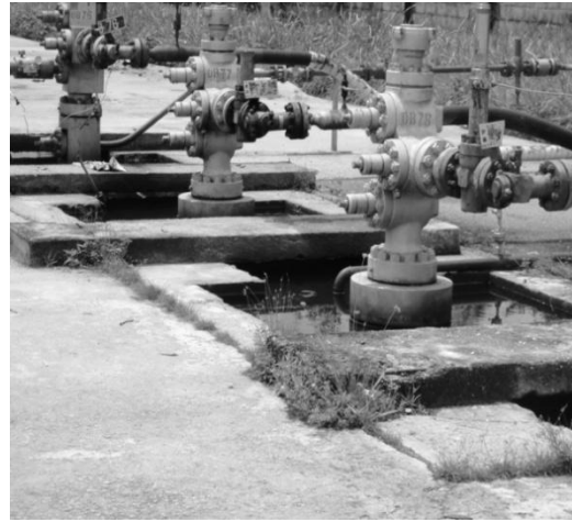
Open Oil Wells with Rusted Oil Well-Heads in Obite
