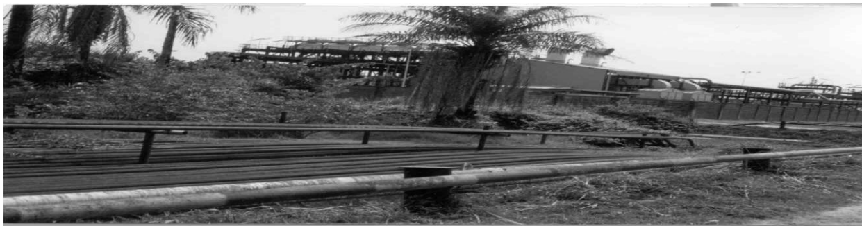
Surface Laid Rusted Oil Pipe Lines in Obagi
