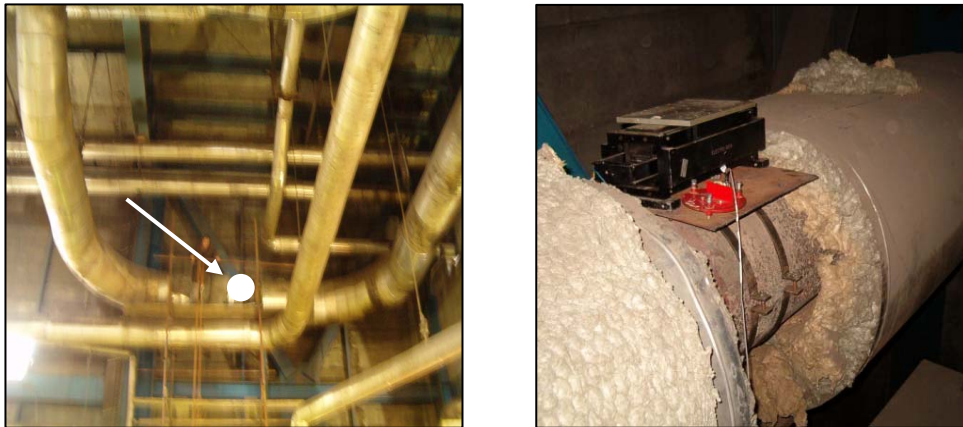
Fig. 6. Position of the shaker on the pipeline
