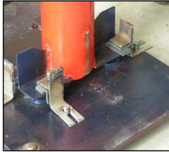
Fig. 14. The limiters at the stop point
