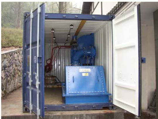
Photo 2: Example of arrangement of the equipment in container SHPP
