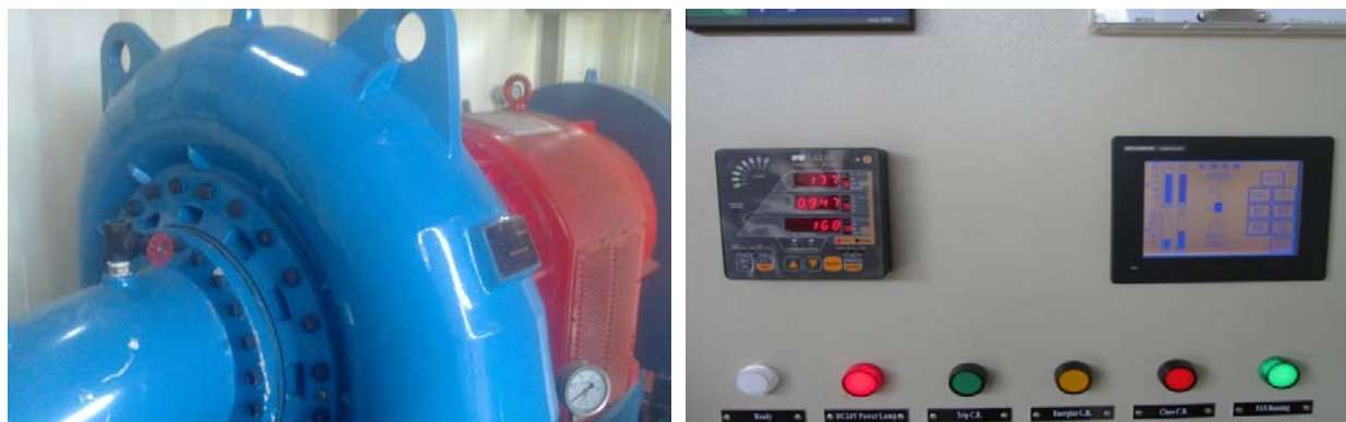
Photo 3: Inside the container during commissioning of MHP Turija 27.06.2013 (177 kVA, 168 kW with 58 m of head and 420 l/sec, it can be seen on the control panel that MHP Turija provided 22 kW more than the guaranteed value of 146 kW at max flow and max head)
