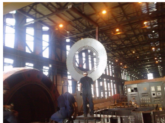
Figure 4. Monolithic end pack of the stator magnetic core in the process of mounting for turbo-generator n.1 in TPP Bitola
