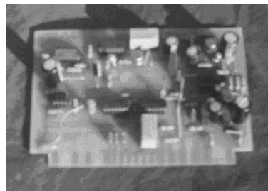
Fig. 5. Practically realized circuit for protection on the excavator
