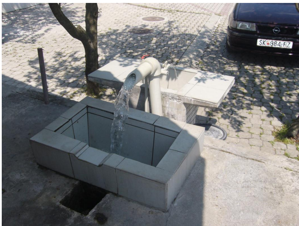
Fig. 4. Artesian drill hole of Raotince site.
