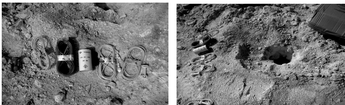
Figure 4 Nonel detonators with booster around drilled hole
