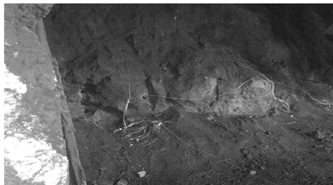
Figure 4. Connecting the blastholes with Nonel system
