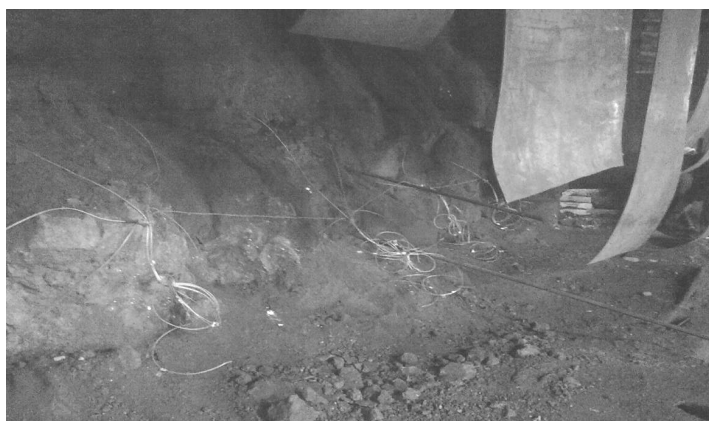
Figure 5. Protection from flying debris with rubber screens
