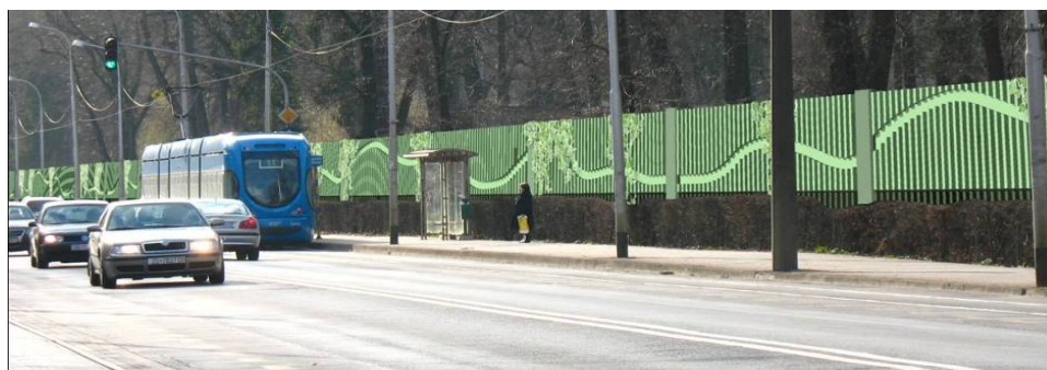
Photography 1: “Ruconbar“ noise protection barrier
