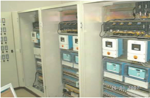
Figure. 3 The control cabinets.
