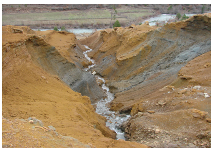
Figure 10. Canyon on the dam Kurbnesh created due to water erosion.
