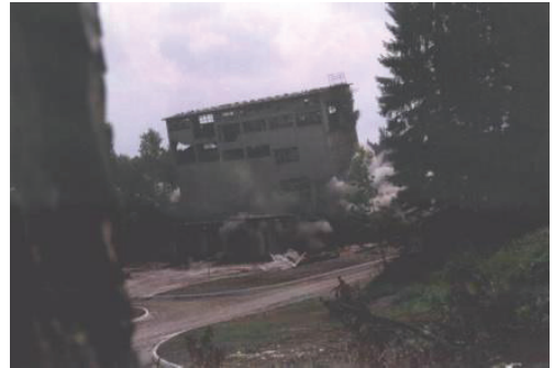
Figure 3. Demolition of the separation unit.
