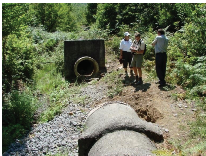
Figure 9. Defect at water diversion channel.
