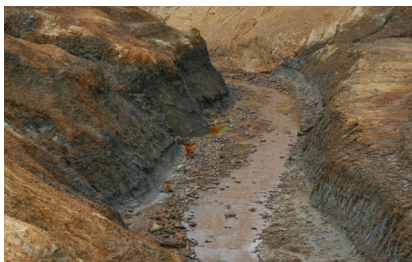
Figure 3. Canyon on the dam nr 1 Fush-Arrez created due to water erosion.
