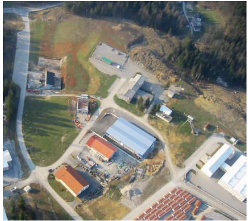
Figure 5. Partially refurbished area of the previous mine in 2005.
