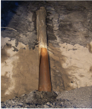
Figure 10. The pipe in the well how it was on the intersection of vertical and horizontal tunnel.
