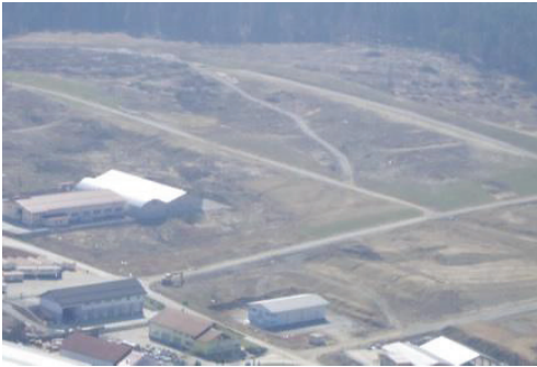
Figure 8. Remediated land above the excavation fields in 2009.
