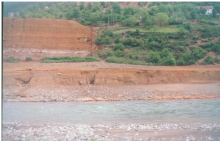
Figure 6. Dam No 4 above and No 2 below in the Small Fani River bed.
