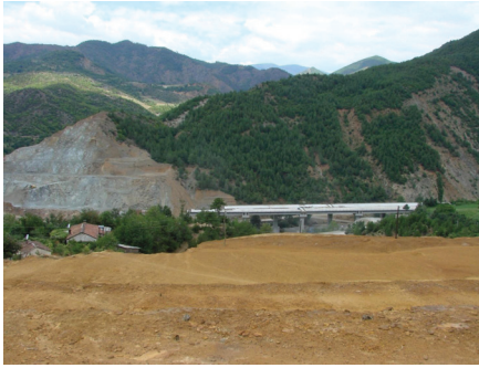
Figure 12. Risk of collapse by the dam of Reps site.
