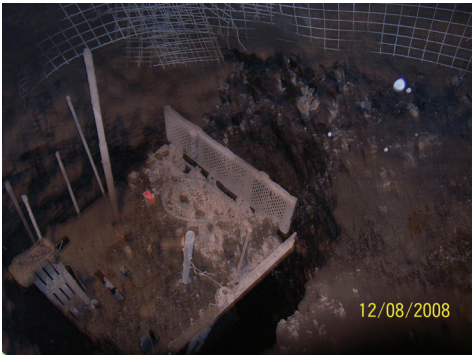
Figure 15. The platform Alimak and the bottom of the vertical shaft – breakthrough.
