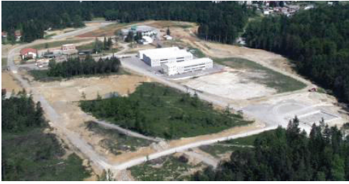
Figure 7. Rehabilitation works above the excavation fields in 2000.
