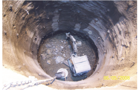
Figure 11. The machine excavation on the bottom of the shaft.
