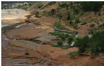
Figure 4. A part of water diversion structures and erosion canyon.
