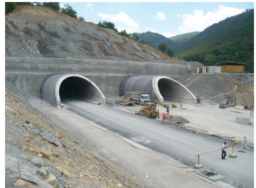
Figure 2. View of the west portal.
