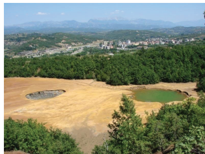
Figure 8. The view of 2 dangerous holes in Resheni dam.
