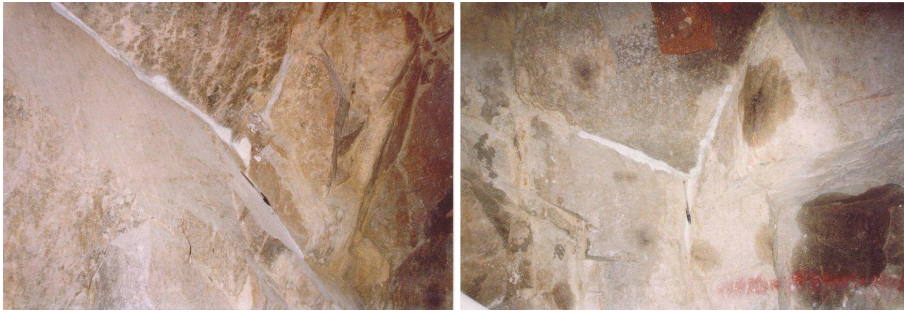
Figure 1. Examples of unstable blocks on the sidewall of an underground excavation.
