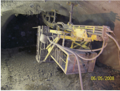
Figure 14. The platform Alimak.
