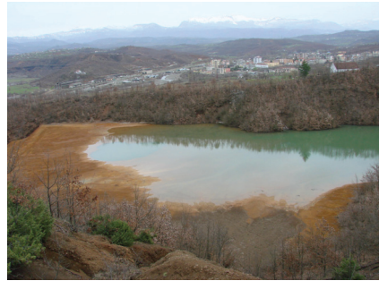
Figure 7. The surface of Resheni dam covered by water.
