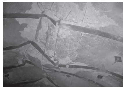
Figure 14. Roof failure of the support.
