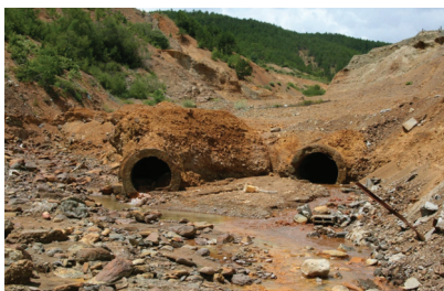
Figure 2. A big part of the dam is damaged due to water erosion.
