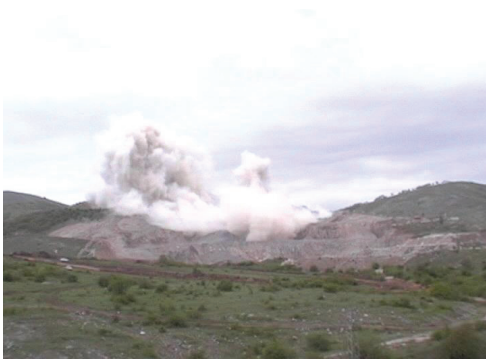
Figure 4. Fragments of the development of the explosion in both sections of the Studena quarry with the explosive ANFO-L.
