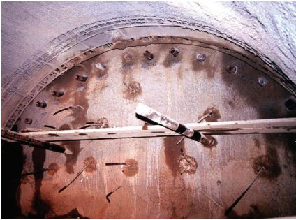
Figure 2. The appearance of tunnel face that is placed Umbrella Pipes and Face Bolts.
