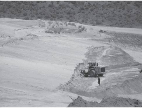
Figure 2. Beginning phase of technical reclamation - slope terracing with a machine.
