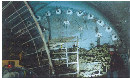
Figure 3. An appearance of the metro tunnel face with umbrella pipes.
