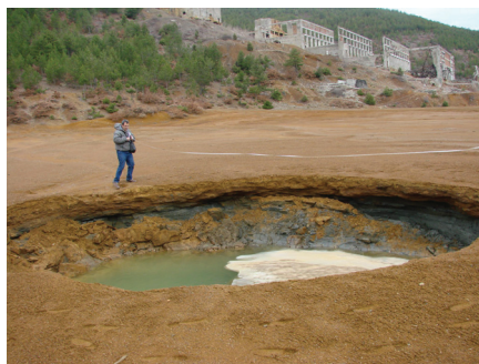
Figure 11. The hole on the Kurbneshi dam.
