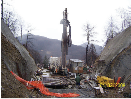
Figure 5. Drilling equipment FRASTE FS400 on the location of vertical shaft.
