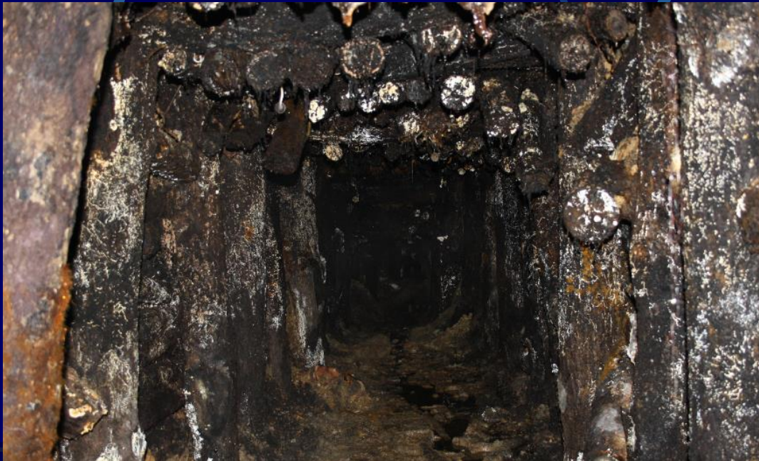
Tunnel at CRVEN DOL (Allchar)
