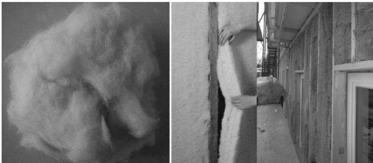
Figure 1: Application of wool for insulation of buildings, [6]
