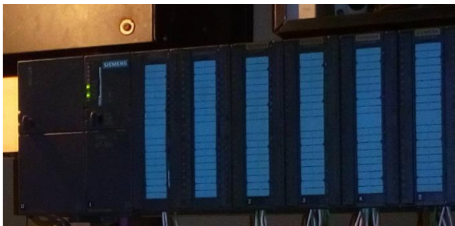
Figure 2: PLC Siemens with analogue cards
