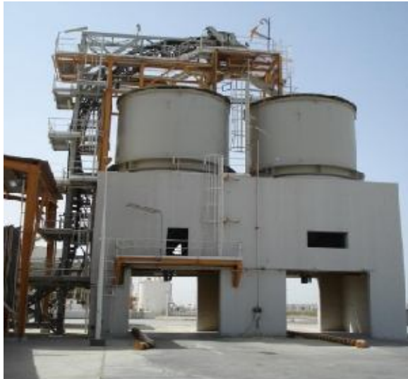
Figure 6: phase 2&3 conveyer to silo
