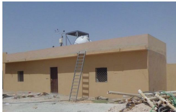
Figure: (2) shows the exterior finishes in test rooms.
