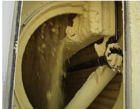
Figure 8: Granulator at the start up
