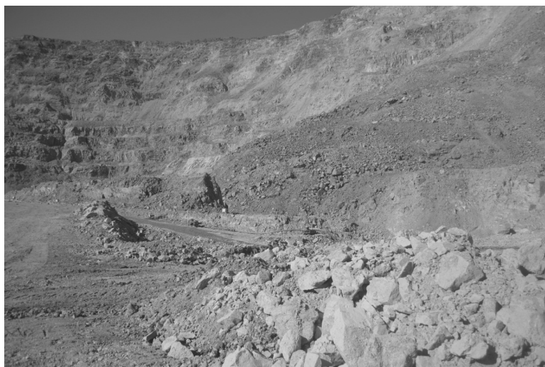
Fig.1 Appeared landslide (view from the north-east)
