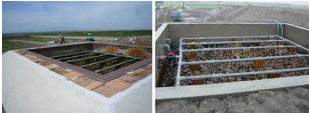
72. (Hashimoto Landfill, Japan) Figure 72. Example of circulation of leachate (Hashimoto Landfill, Japan)
