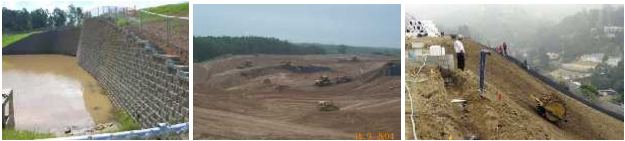
Figure 18. Construction of retaining facilities on the sanitary landfill
