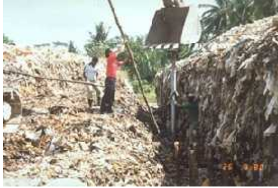
Figure 9. Setting the piles using a backhoe (Ampang Jajar Landfill, Malaysia)
