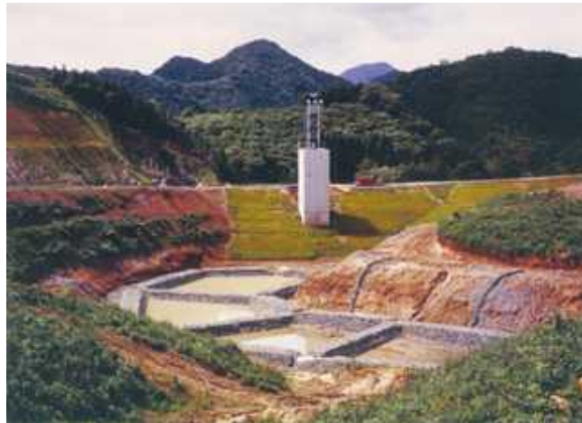
Figure 32. Method of pit-pump of leachate (Busetsugaura landfill, Fukuoka-Japan)
