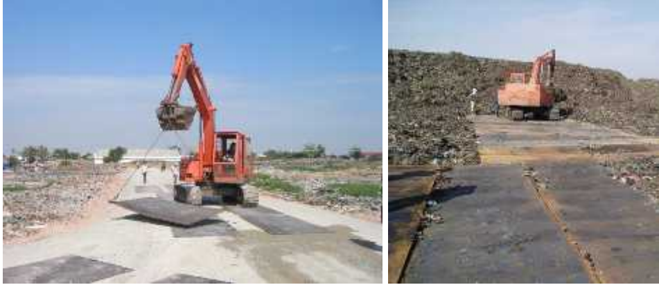
47. Figure 47. Measures of protection with steel plates
