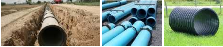
23. Figure 23. Construction of drainage with drainage ditch
