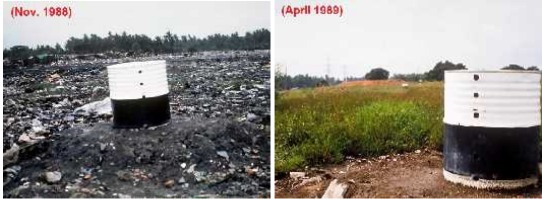
Figure 96. Measure 3 - Ventilation and stabilization of landfill (Ampang Jajar Landfill, Malaysia)
