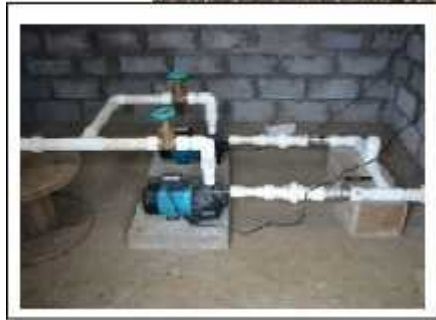
73. ( ) (Tafaigata landfill, Samoa) Figure 73. Circulation pit (Tafaigata landfill, Samoa)
