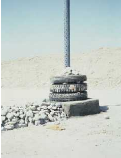
Figure 15. Example of the use of used tires as material for protection of the ventilating pipe (Kahrizak Landfill, Tehran-Iran)
