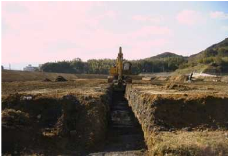
Figure 64. Trench extraction wastewater for the normal flow of air from the landfill layer (China: City of Weifang, Shandong Province)
