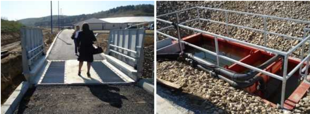
Figure 84. Facility for washing and disinfecting vehicles
