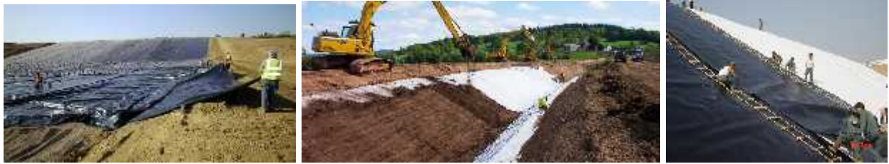
19. Figure 19. Construction of liner facility on the sanitary landfill
