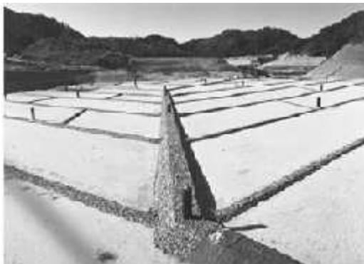
Figure 40. Good example of leachate collection facilities and good example of main leachate collection pipe
