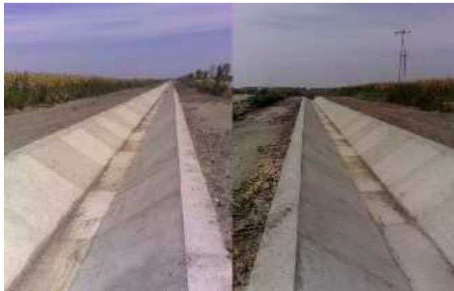
22. Figure 22. Perimeter drainage of the sanitary landfill
