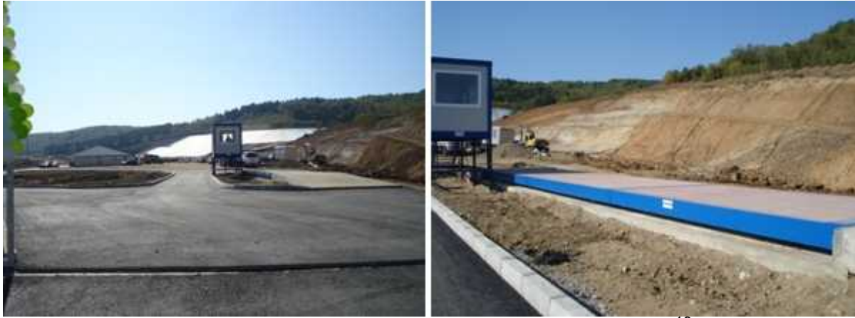
Figure 83. Weighbridge on sanitary landfill
