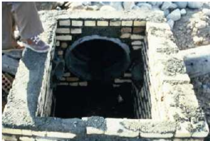
Figure 14. Example of using bricks and making sump for collecting leachate (Kahrizak Landfill, Tehran-Iran)
