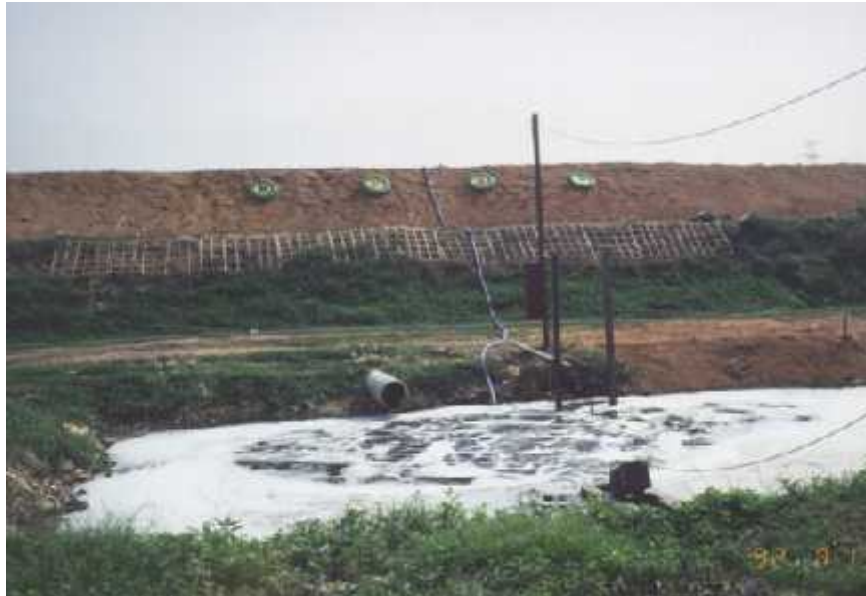
Figure 31. Method of natural flow of leachate (Ampang Jajar Landfill, Malaysia)
