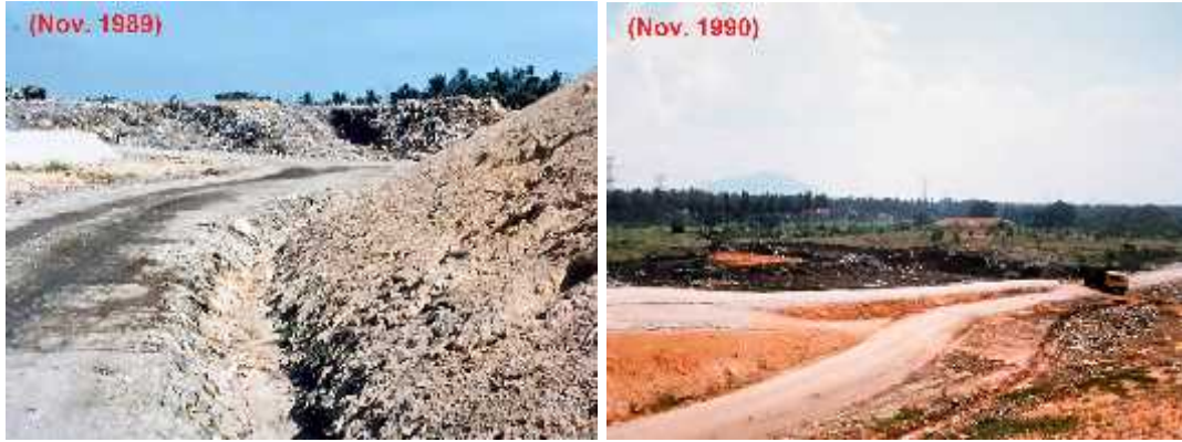
Figure 95. Measure 2 - Access road and drainage channels (Ampang Jajar Landfill, Malaysia)
