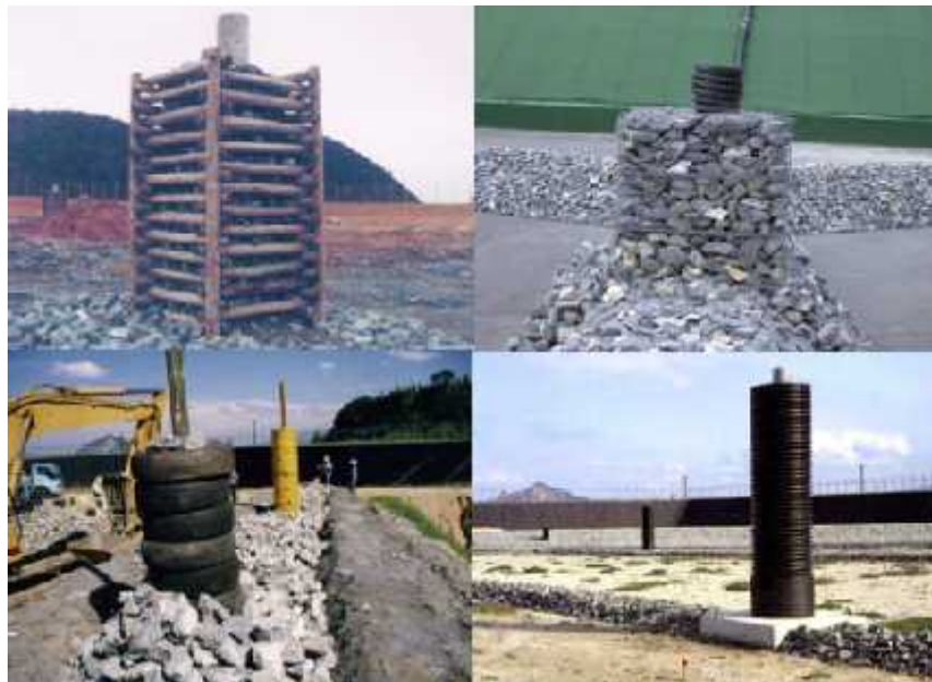
Figure 61. Types of construction of vertical ventilation pipes
