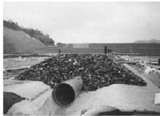
Figure 40. Good example of leachate collection facilities and good example of main leachate collection pipe
