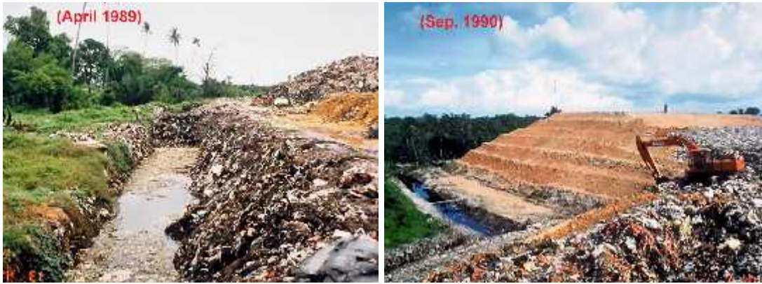
97. 4 - (Ampang Jajar , ) Figure 97. Measure 4 - Trenches and embankments of landfill (Ampang Jajar Landfill, Malaysia)
