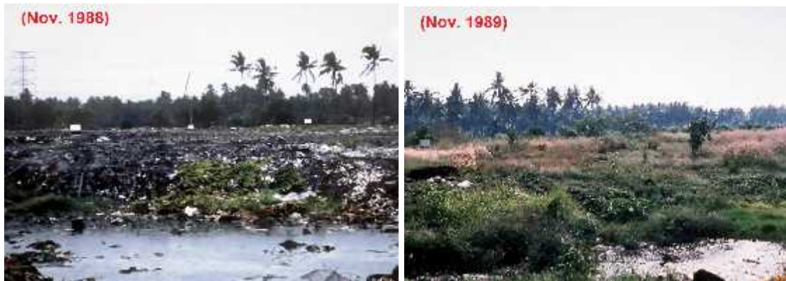
94. 1 - (Ampang Jajar , ) Figure 94. Measure 1 - Covering the soil cover (Ampang Jajar Landfill, Malaysia)
