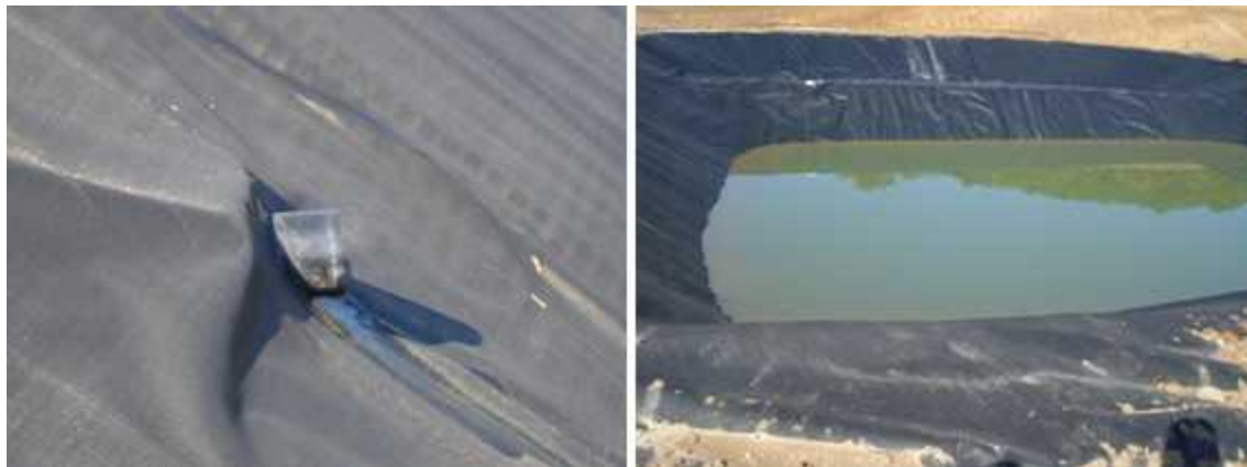
Figure 27. Open discharge pipe of leachate in to the retention pit
