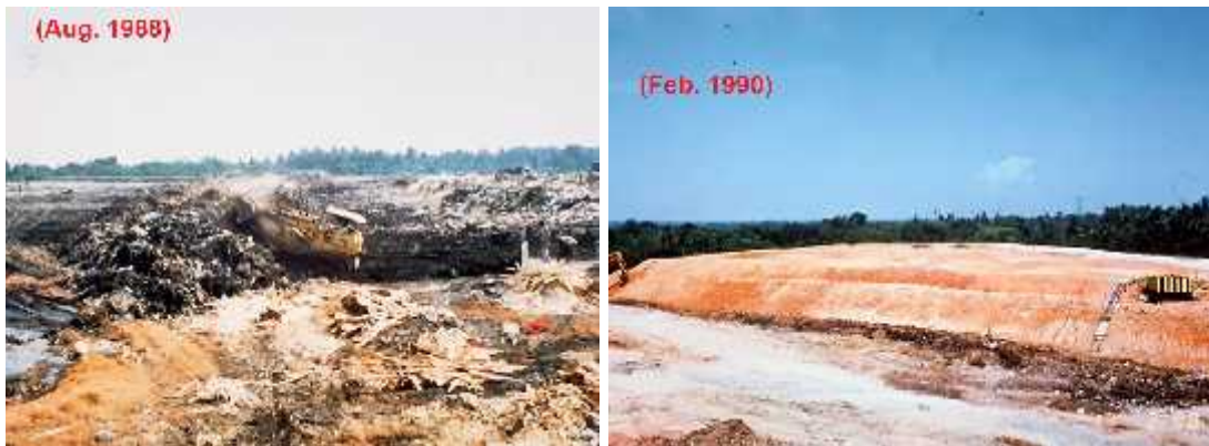
98. 5 - (Ampang Jajar , ) Figure 98. Measure 5 - Retaining embankments and slopes of landfill (Ampang Jajar Landfill, Malaysia)
