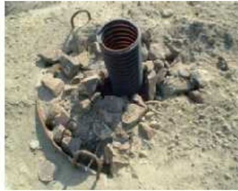
Figure 60. Bad examples for the operation of ventilation pipes (when waste is crowded and when pipe is buried)
