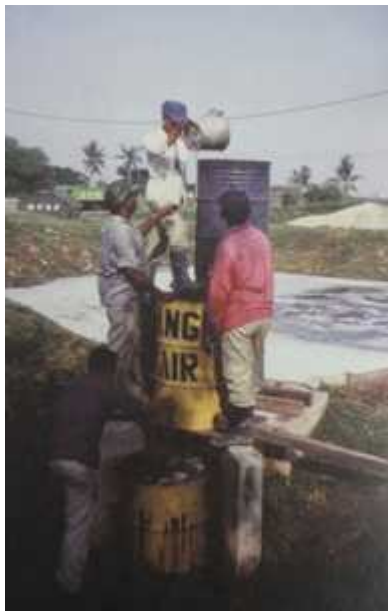
Figure 104. Installation of the system for physical treatment of leachate (Ampang Jajar Landfill, Malaysia)
