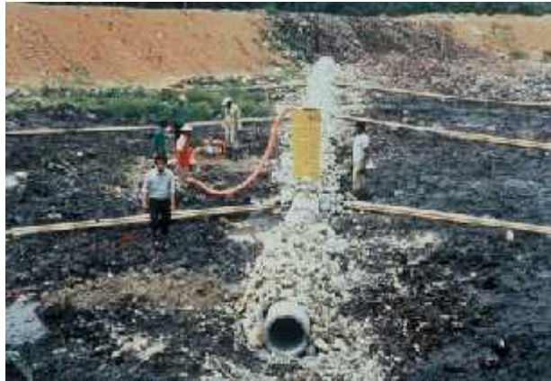
Figure 13. Example of the use of bamboo as a pipe for collecting the leachate (Ampang Jajar Landfill, Malaysia)
