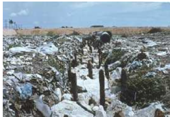
Figure 9. Setting the piles using a backhoe (Ampang Jajar Landfill, Malaysia)
