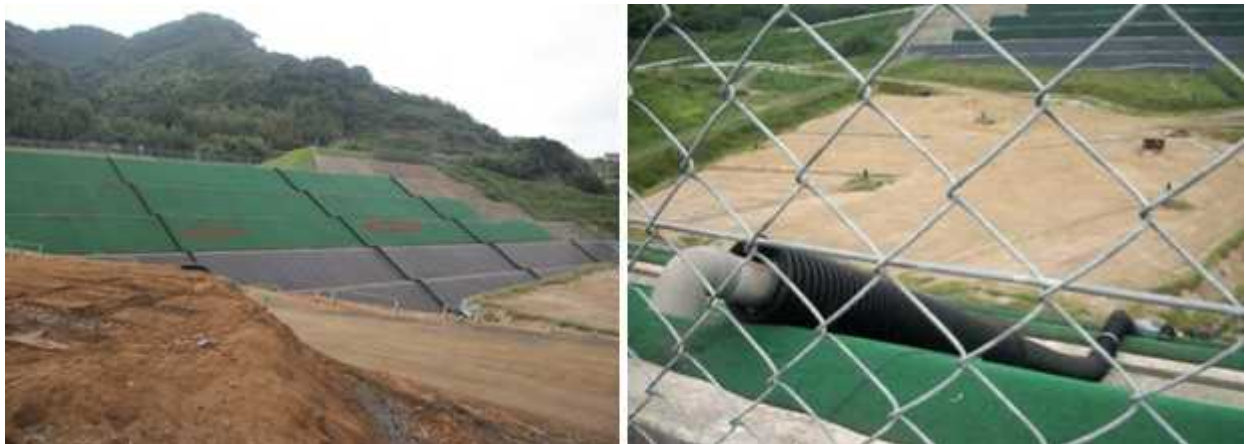
51. (Nakata , - ) Figure 51. Installation example of inclined gas venting pipes (Nakata Landfill, Fukuoka-Japan)
