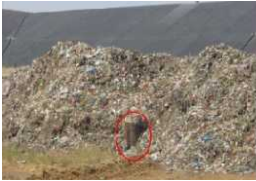
Figure 60. Bad examples for the operation of ventilation pipes (when waste is crowded and when pipe is buried)
