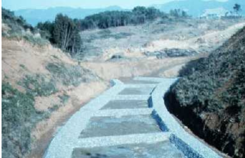
Figure 37. Placement example of leachate collection discharge pipes (Busetsugaura landfill, Fukuoka-Japan)
