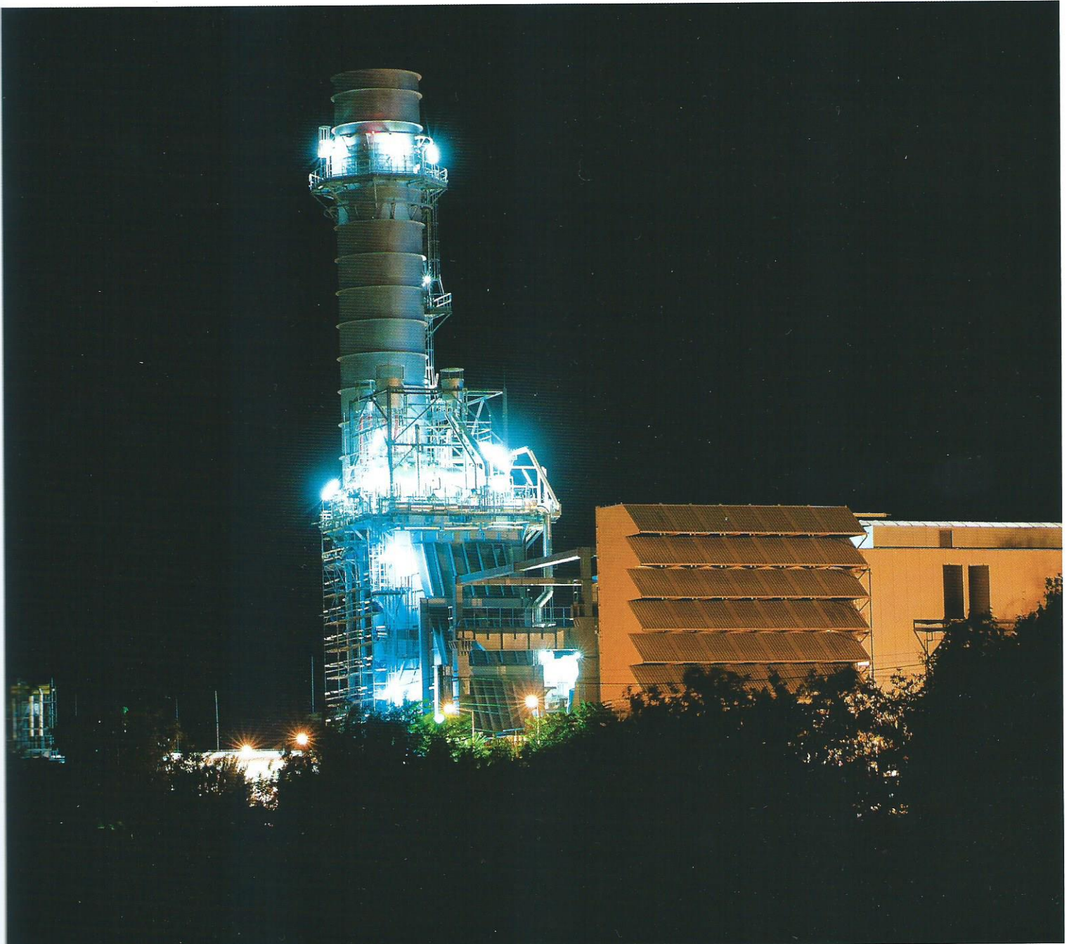
Te-To, electric power and heating plant, Skopje
