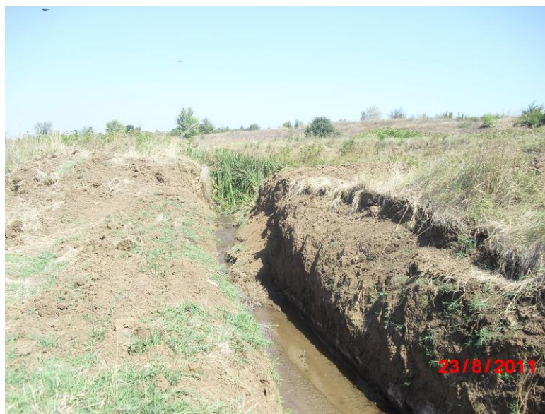
Figure 10. Canal for irrigation/drainage in the project location (because of the project construction the existing canal is attached to the temporarily excavated channel)
