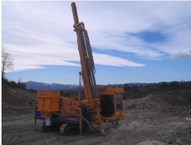
Figure 2. Machines for drilling HBM 120
